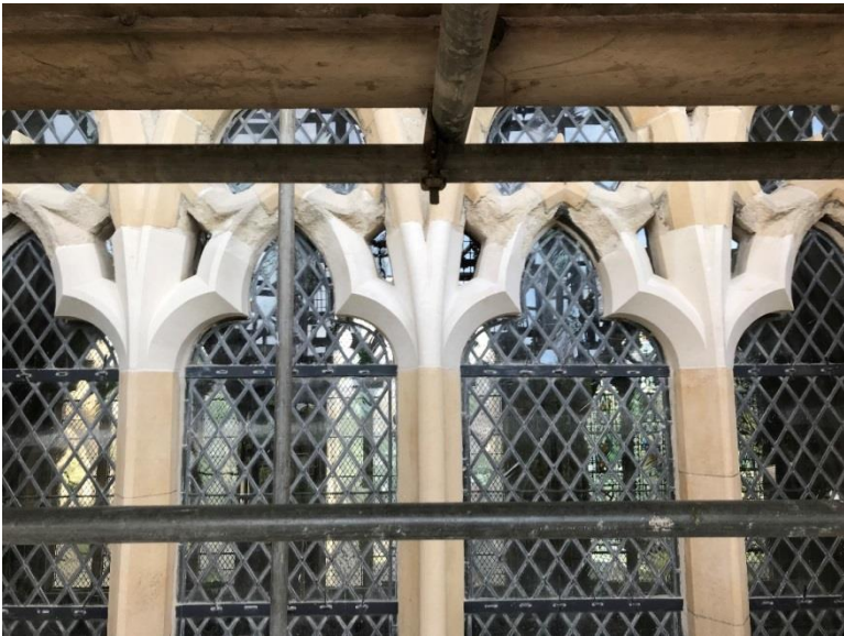
New Tracery springer stones in Beer stone Bay 11 South Quire Clerestory
