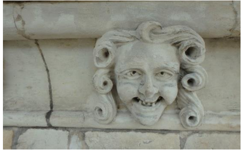
Carved corbel after cleaning and repair
