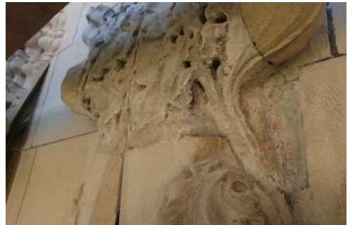
Blind tracery carved finial after cleaning revealing Medieval paint fragments on close inspection
