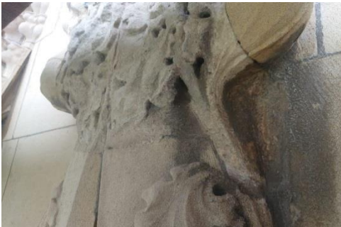
Blind tracery carved finial with sulphation prior to cleaning
