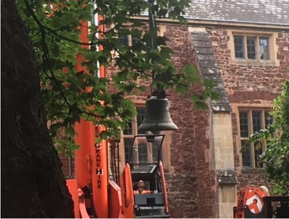
With the Cathedral bells having now been silent for over two months, we are starting to near the end of the bell refurbishment project. On Saturday 4<sup>th</sup> August, a second crane lift returned our two treble, or lightest, bells back home to the belfry, having undergone their maintenance work at Taylors bell foundry in Loughborough.
